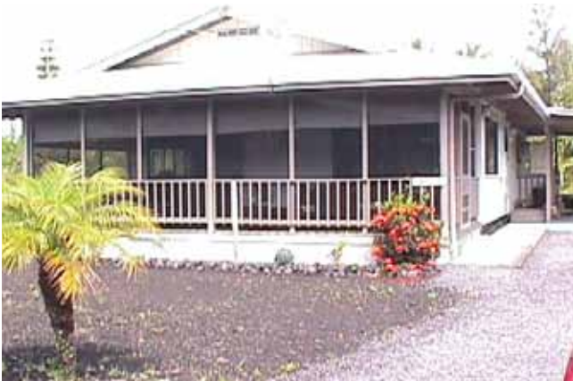
The front of this house is a lanai (interior view at right) built over a solid concrete tank. While high-priced, solid-pour concrete tanks such as this offer attractive architectural design options.
