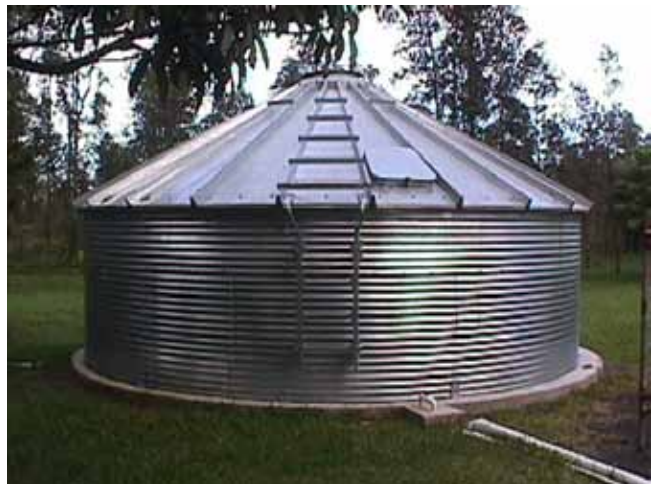
Some corrugated tanks have solid covers. This model has a top hatch for access and a liner secured to the sides with bolts.
