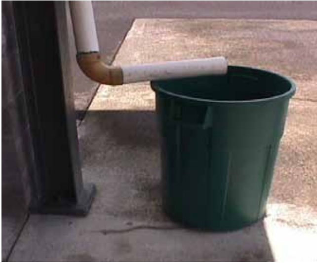
Water collected and held in containers that haven't been approved for water storage can be deadly. Plastic garbage containers, for example, can contain toxic dyes and biocides that could leach into the water.
